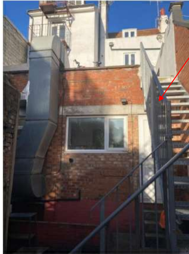
Stairs to existing dwelling
